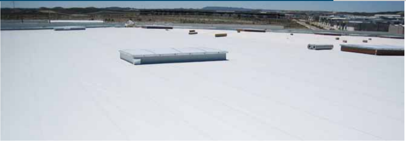
Spain , Zaragoza, Aceros IMS plant
