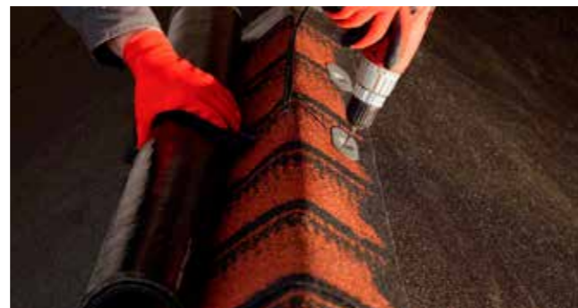
Mechanical fixings along ridge and selvage overlaps
